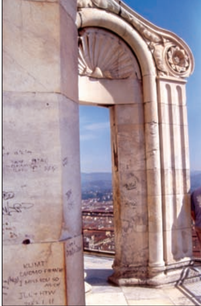
LEFT: The lantern at the top of the dome has eight hollow buttresses that line up with the eight ribs. The lantern acts as the common keystone.
