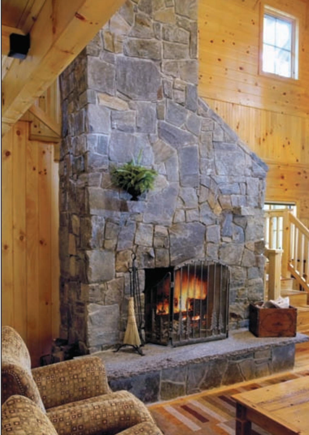
ABOVE: American granite mosaic pattern shaped by mason on site.
