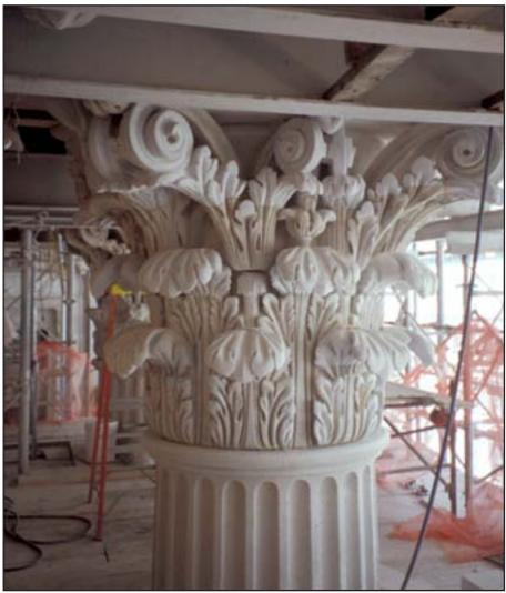
ABOVE: The Chambers Street portico columns capitals during restoration. Craftsman anchored the newly carved sections to the original capitals using stainless-steel pins and epoxy adhesive.
