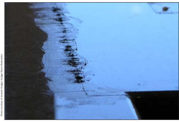
RIGHT: Here a Galaxy Black Granite top is repaired with the aid of copper shavings, six shades of black tinted adhesive, a cup wheel, slow RPM grinder as well as converted layered and top polishing techniques. The top polish maintained the same reflection of the rest of the surface and displayed the same characteristics of the natural stone.
