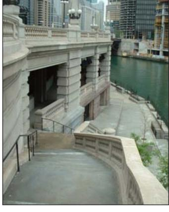
became the material of choice. After some extensive research, site visits and analysis of the original materials, Cold Spring Granite found three finish "recipes" that had a good visual match and characteristics comparable to the original. The restored and new stone appear to blend seamlessly.
