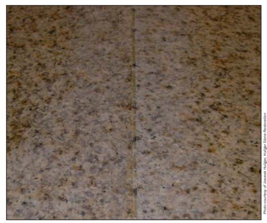
LEFT AND BELOW: The application of adhesive polished flush makes a smooth repair to this stone.
