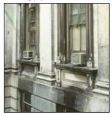
ABOVE: Window and wall details before restoration. Many of the marble decorative elements had been converted to gypsum by exposure to atmospheric pollutants and needed to be replaced by new stone.
