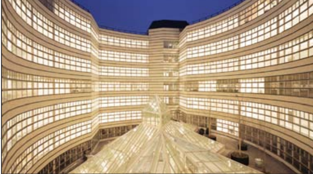
ABOVE: Fredrickstadt Passagen, Berlin, office/retail/apartment complex exterior at night.
