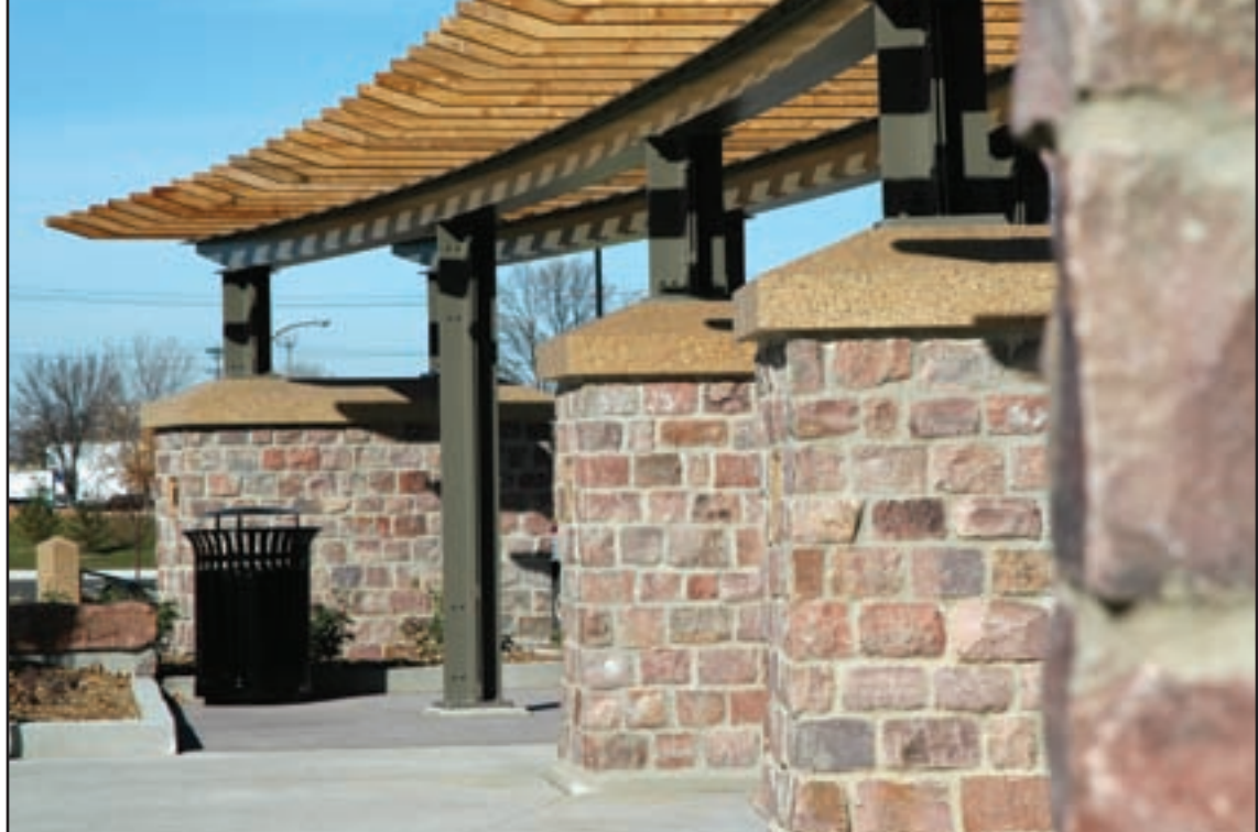
Photo courtesy of Craig Dewitz/Brian Clark & Associates
