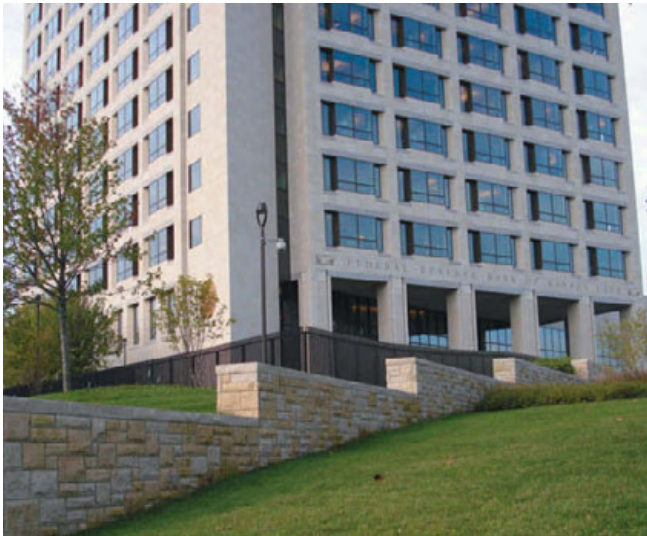
Built of Cottonwood Falls and Silverdale limestone, a low wall surrounds most of the Federal Reserve Bank of Kansas City and pairs nicely with the building's limestone exterior. Photo courtesy of the Building Stone Institute
