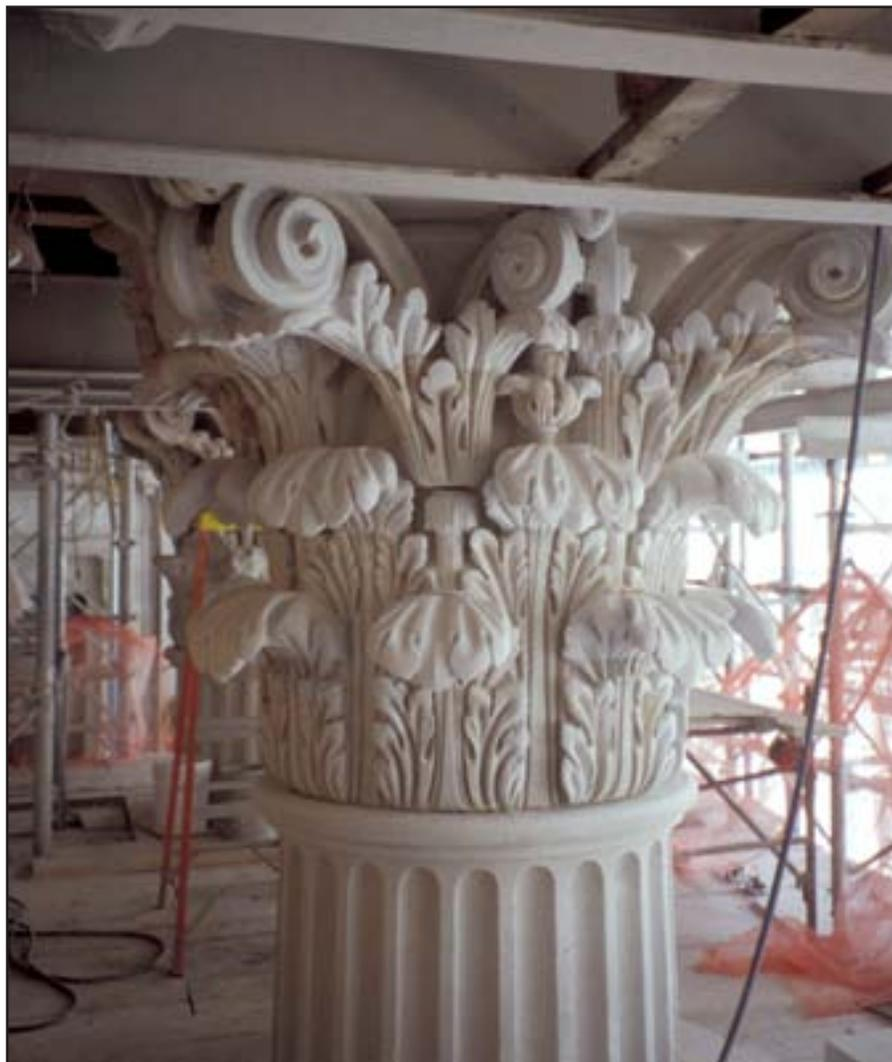
The courthouse renovation included its 30 monumental courtrooms. Stripping 100 years of paint – up to 18 layers – revealed unexpected detailing in the ornamental cast iron and multi-colored patterns on the brick walls. Original paint schemes and marble and glass-tile floors popped into view throughout the building. New York has added the Tweed Courthouse interiors to its own list of historic landmarks.
