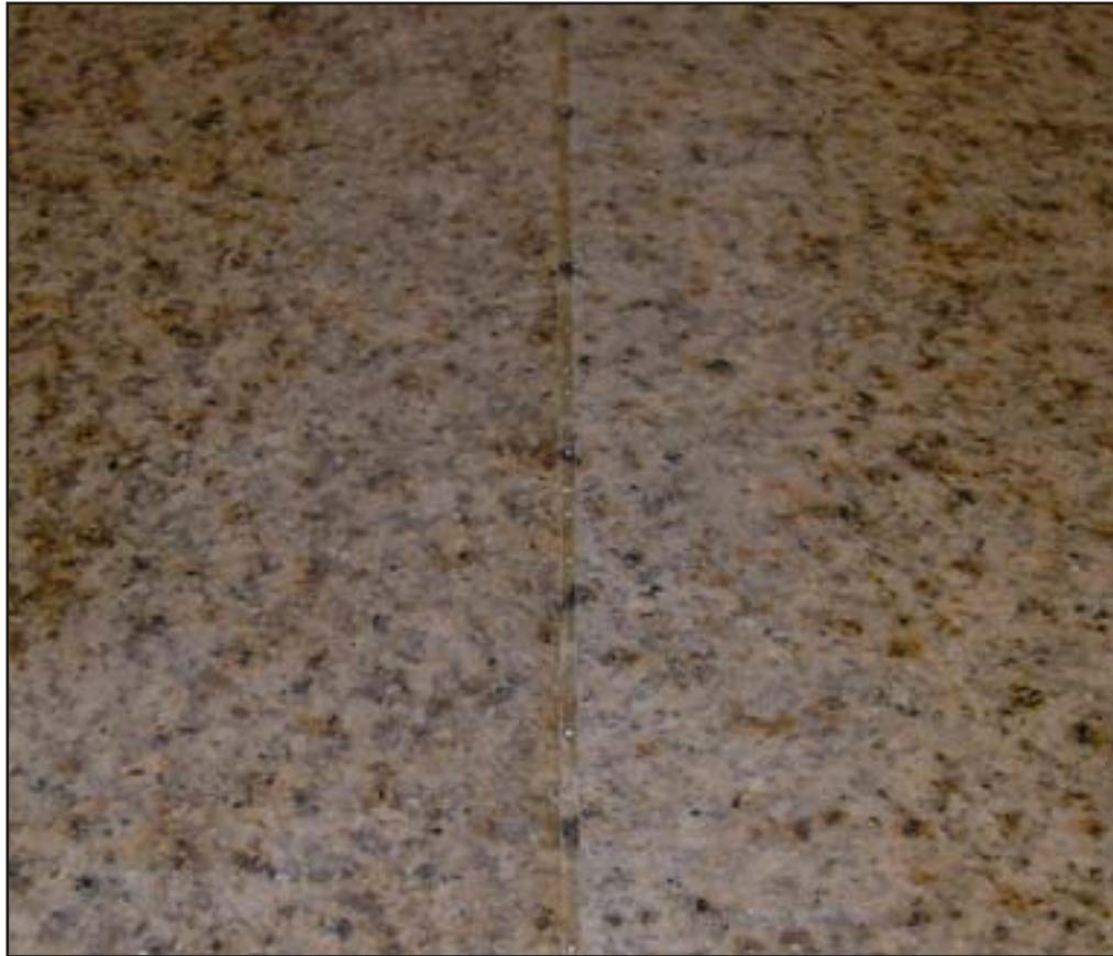
LEFT AND BELOW: The application of adhesive polished flush makes a smooth repair to this stone.
