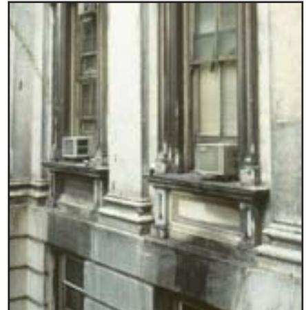
ABOVE: Window and wall details before restoration. Many of the marble decorative elements had been converted to gypsum by exposure to atmospheric pollutants and needed to be replaced by new stone.
