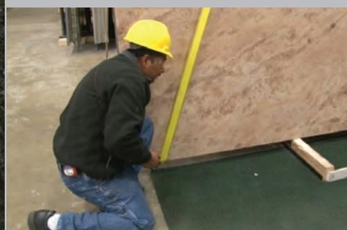
*Attaching a nylon strap to slab*
