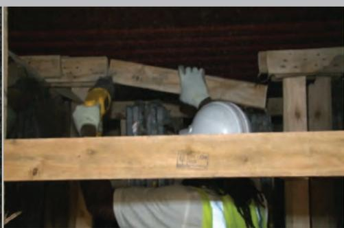
*Worker removing braces from a closed-top container*
