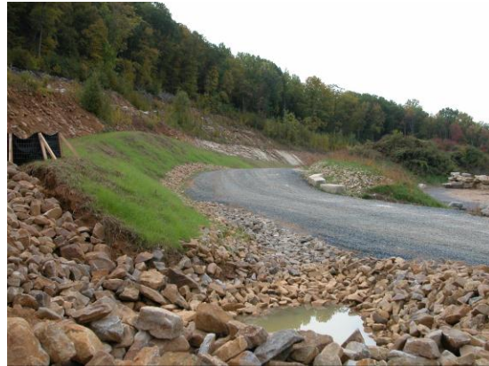
Quarry roads are laid with gravel to minimize dust, and scrap stone is used to create drainage ditches as well as provide support to the adjacent hillslope.
