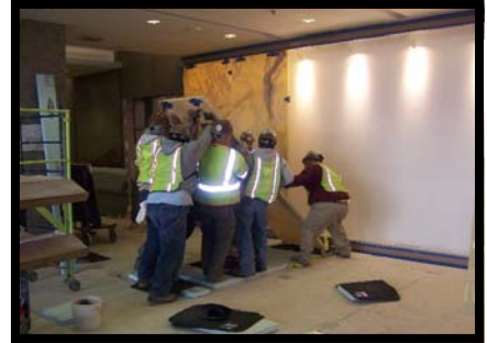
Photo 19: Tilting Laminated Panels of Honey Onyx Into Place
