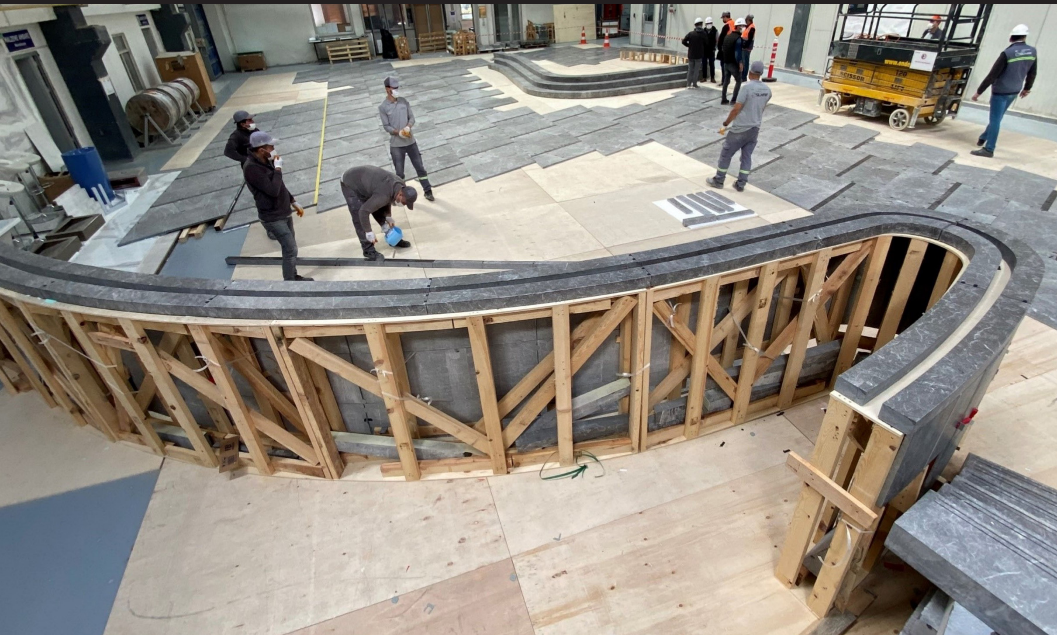
Unprecedented levels of fabrication followed a thorough, 100% dry-lay review process, including all dimensional stones, curving slabs, and the grand stair dry-set in relative position.
