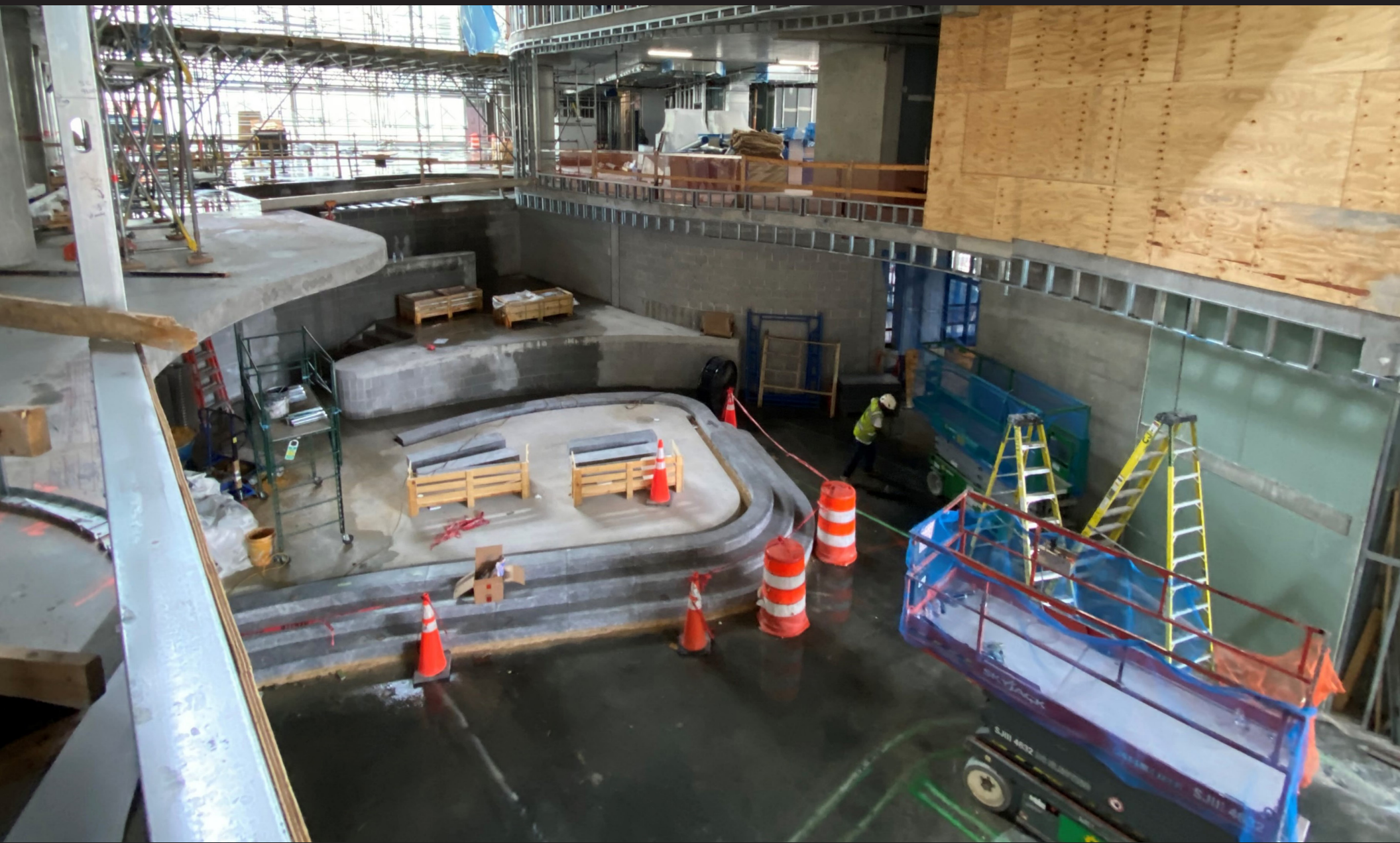
The most challenging parts to finish were the ramp and grand stairs walls. Select mitigations proceeded after a careful review of additional mockups and input from the installers, architects, and owners.
